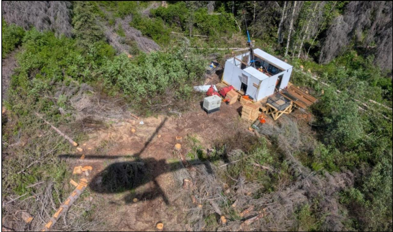
Figure 1 Rig 1 at Whistler located over the Raintree North target area.
